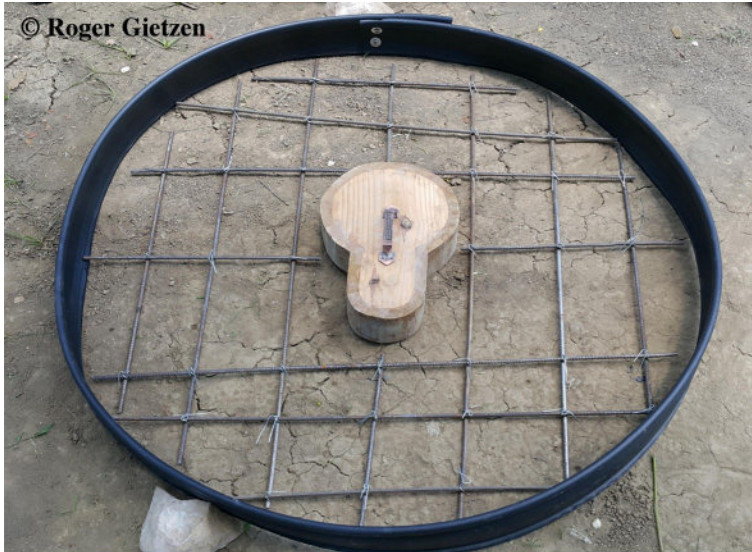
Round form with rebar layout and keyhole form
