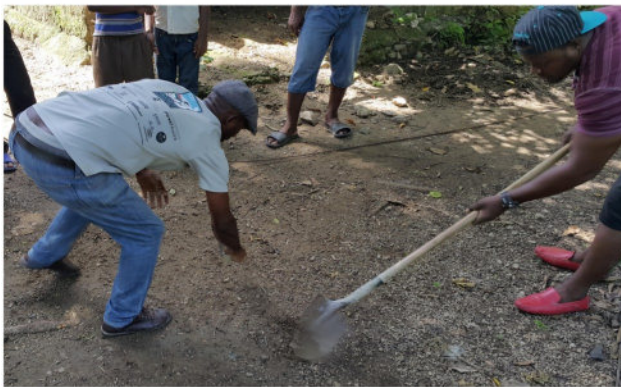
Clean the ground of debris before mixing cement
