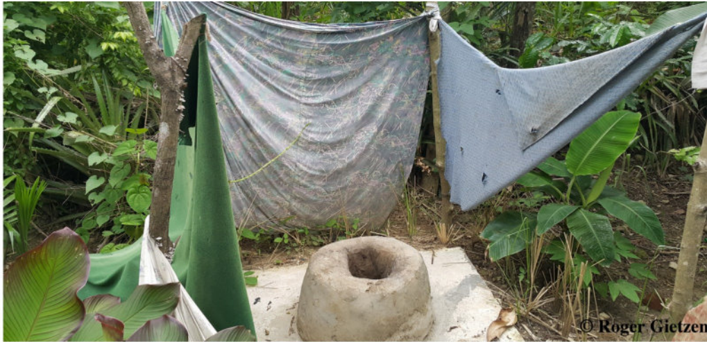
This family built a shelter to enjoy privacy from day 1. Be sure the vetiver grass is not covered by the shelter. Notice here an elevated seat made of concrete.
