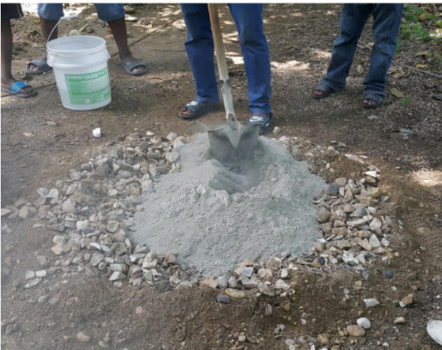
Mix sand, gravel and cement
