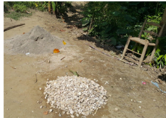
6 buckets of gravel and 2 buckets of sand
