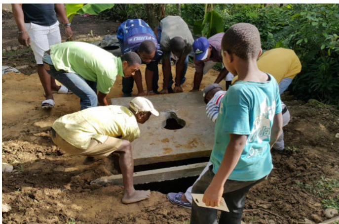
Square slab being moved to final position
