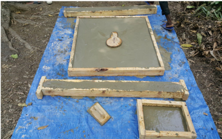
Square slab, cap and beams poured and in forms
