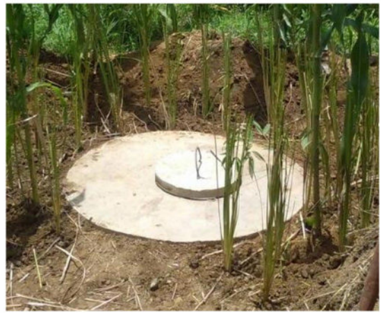
Round slab in final position
