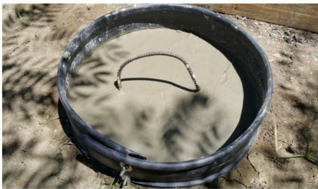
Round cap with rebar handle
