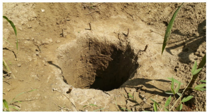
Round pit dug to match round slab
