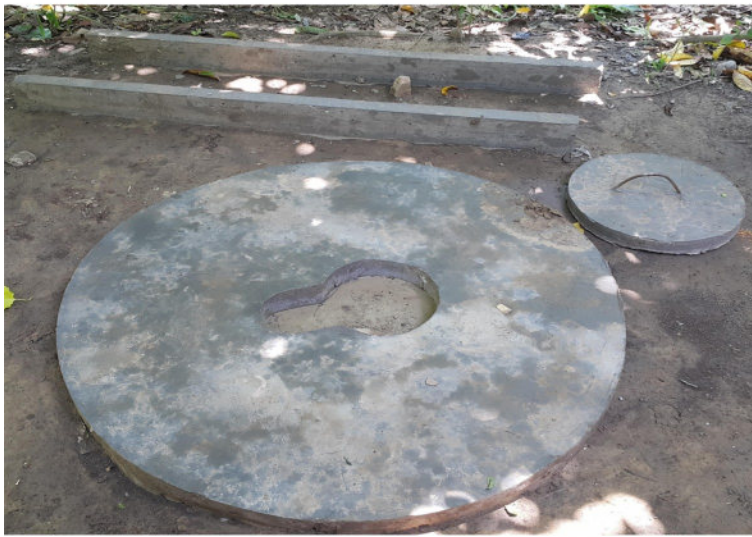
Round slab, cap and beams
