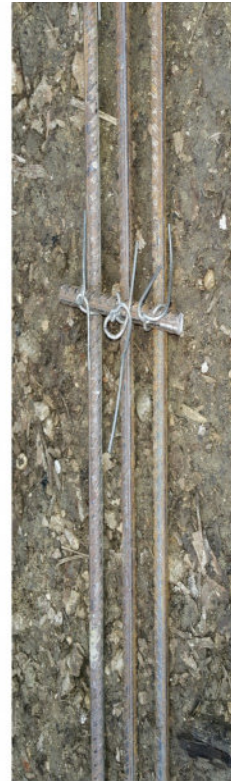
Beam rebar layout
