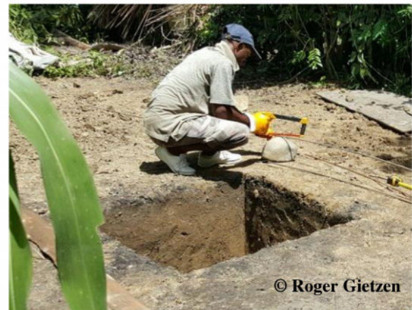
Square pit dug to match square slab
